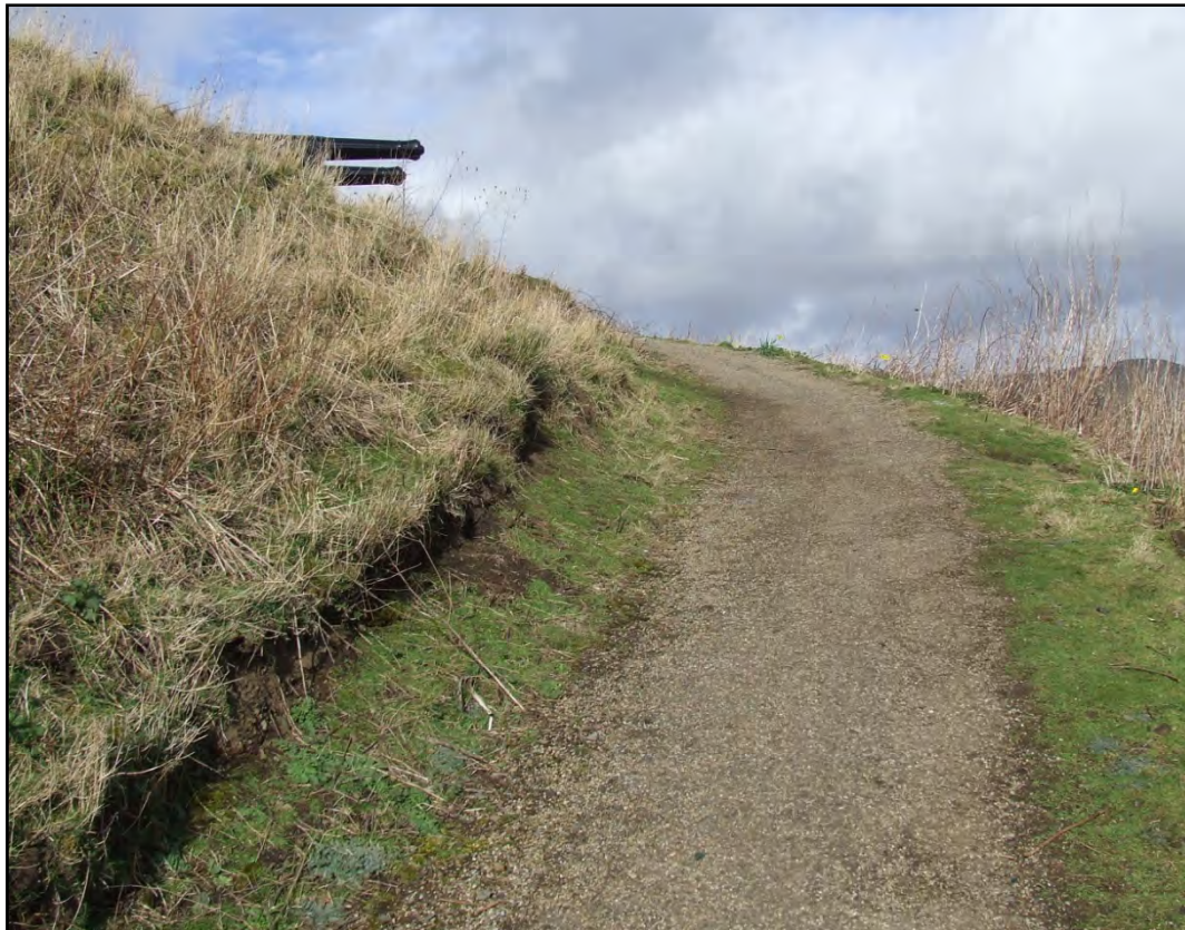
Figure 13: Path bulldozed through the ramparts of the Iron Age fort. (Photo: JGH).
