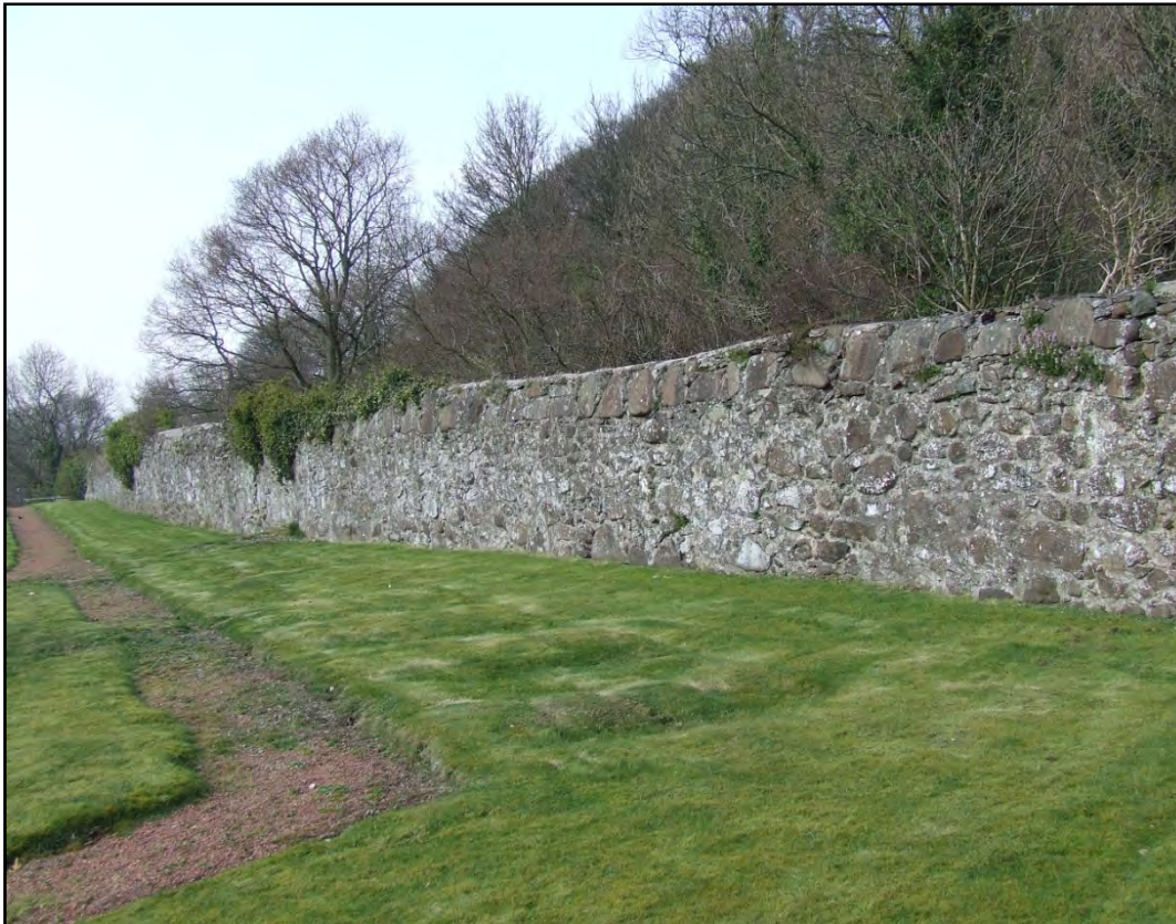
Figure 15: Park Dyke at St Thomas Cemetery; note the massive stones just below the top and the absence of a formal coping.
