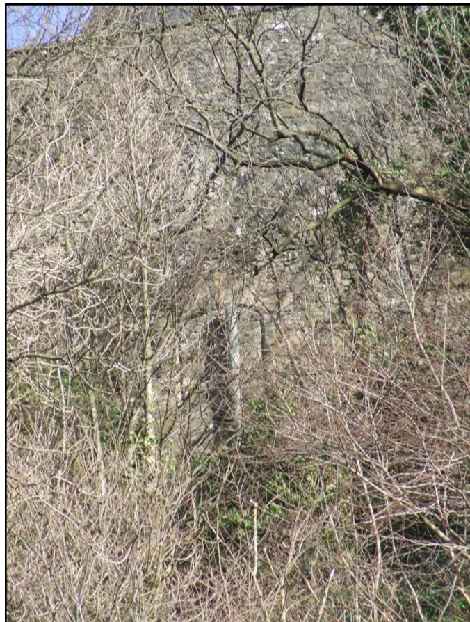
Figure 4: The southern postern as seen from the Low Back Walk; the Outline surrounds the pipe; the slope is too steep and dangerous for a closer shot. (Photo: JGH).
